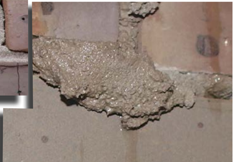
Fig. 2 - Soaked Mortar On Inside Of Wall
