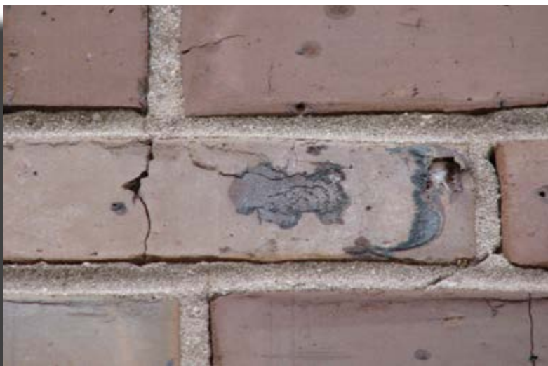
Fig. 1 - Broken Brick & Open Mortar Joints
